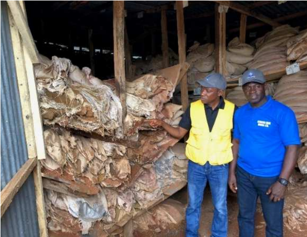
Before = KCM's sample shed in need of attention.
